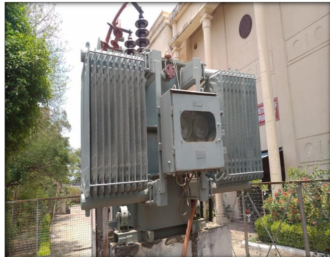
Fig.2.1 Transformer (500 KVA) at 33 KV Sub-station
