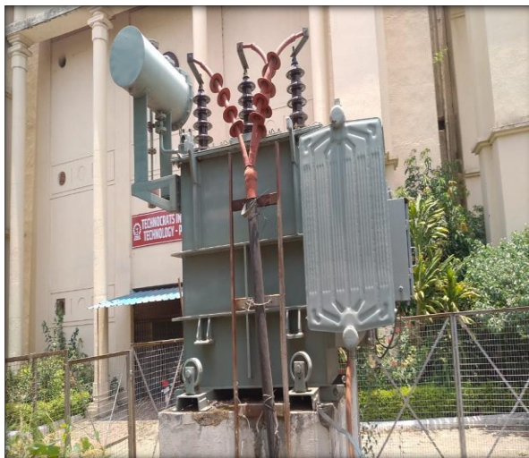
Fig.2.1 Transformer (500 KVA) at 33 KV Sub-station
