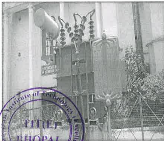
Fig.2.1 Transformer (500 KVA) at 33 KV Sub-station Anand Nagar, Bhopal
