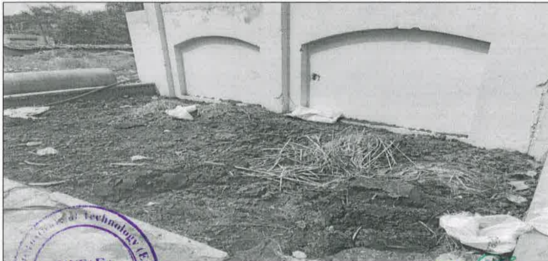
Figure 4.3 Compost pit in the institute campus
