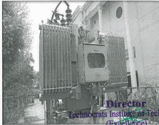
Fig.2.1 Transformer (500 KVA) at 33 KV Sub-station Anand Nagar, Bhopal
